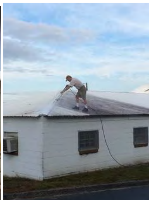
Pressure washing the roof
