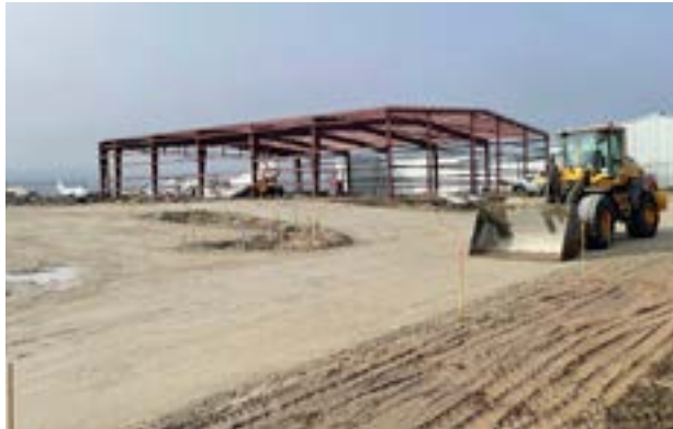
Event Center under construction
