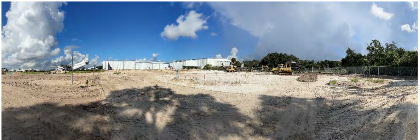
Event Center construction site showing current progress.
