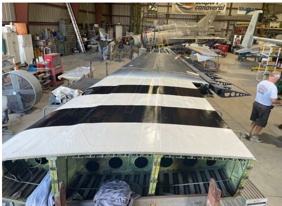
Refurbished C-47 wing to be used as an overhead canopy at the new Event Center
