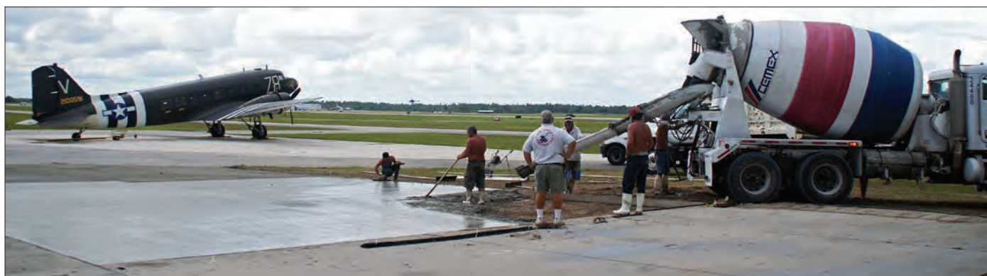
Finishing the concrete pour in front of the restoration hangar
