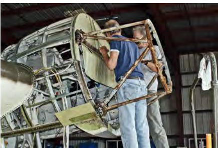
Norm Daniels and Al McQueen work on C-47 nacelle repair.
