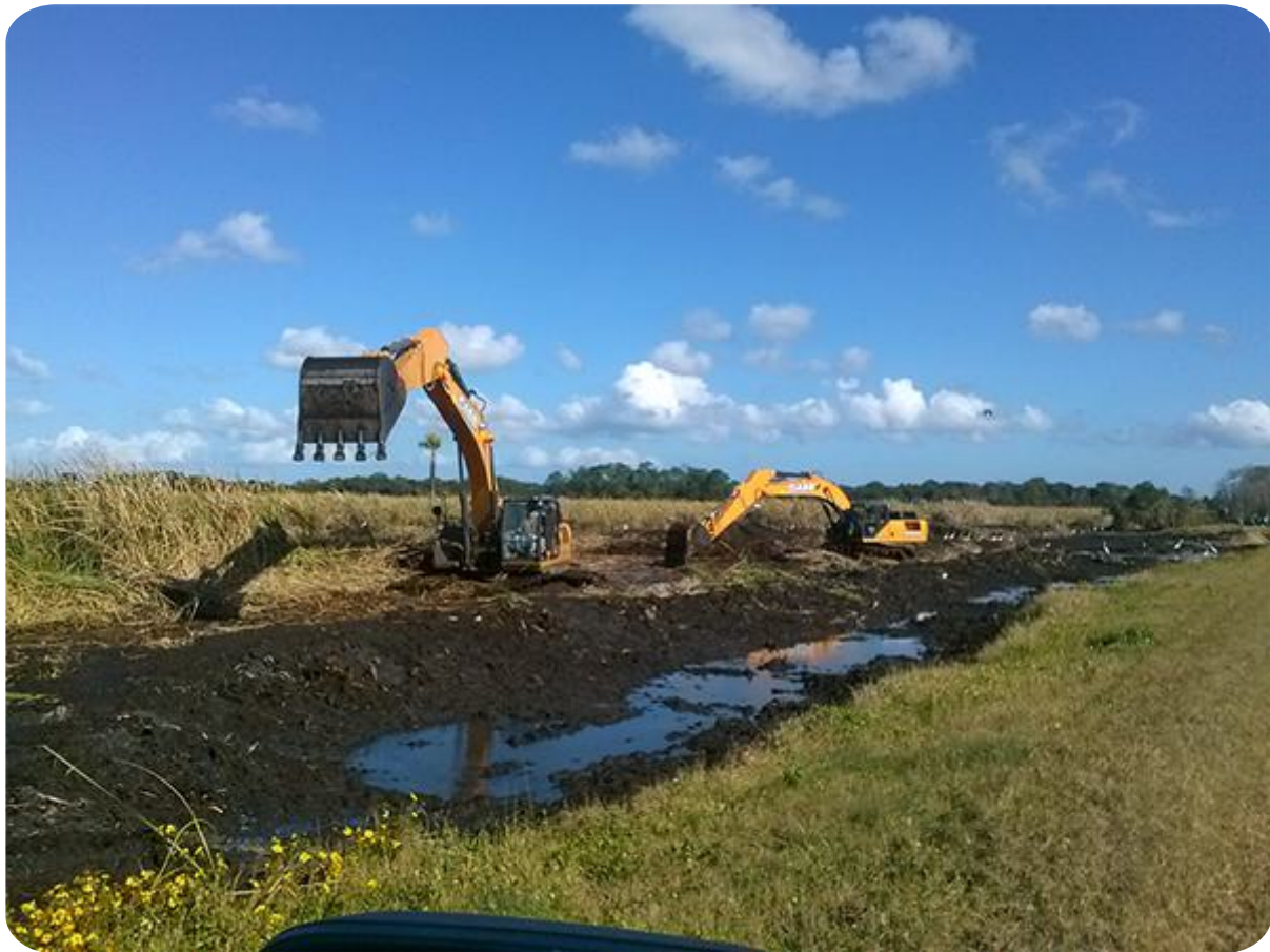
Demucking project at the Orlando Wetlands
