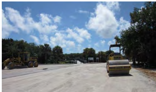
Busy at work paving new road! Photo by Candice Stevenson
