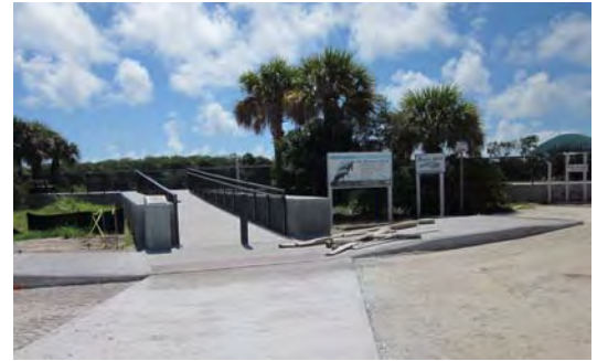
Sidewalk improvements at the observation deck. Photo by Candice Stevenson
