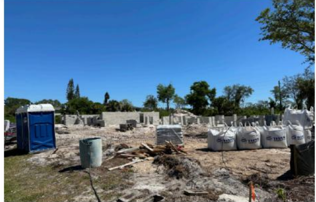
Several multi-family quadruplexes are under development on Fox Hollow Drive.
