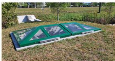
Left: The new baffle box in Sand Point Park with its clear top.
